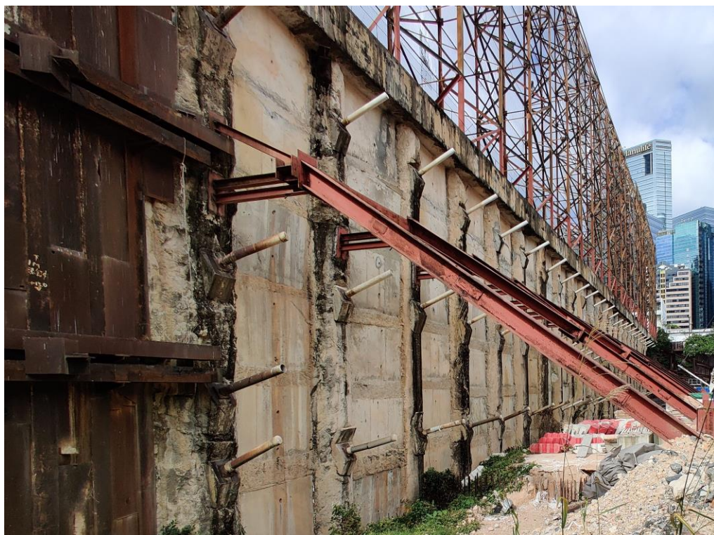
Plate 4: General View of the Bored Pile Wall
