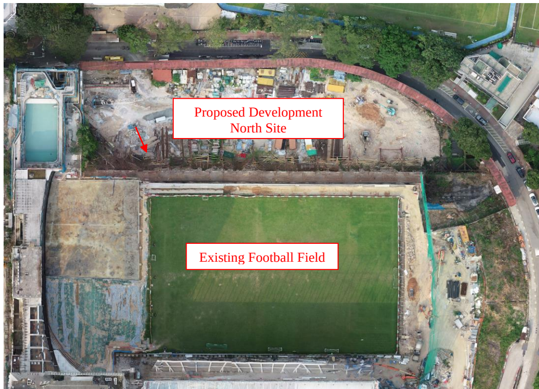
Plate 1: Top View of the Site
