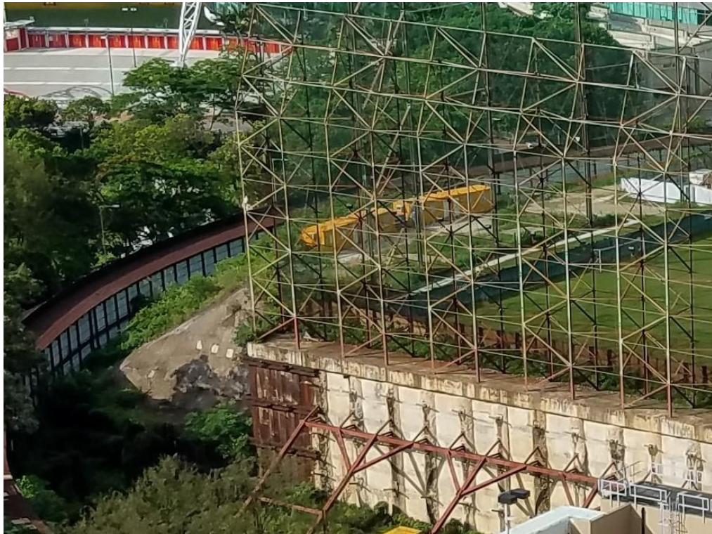
Plate 3: General View of the Southern End of the Site and the Existing Slope 11SW-B/C659
